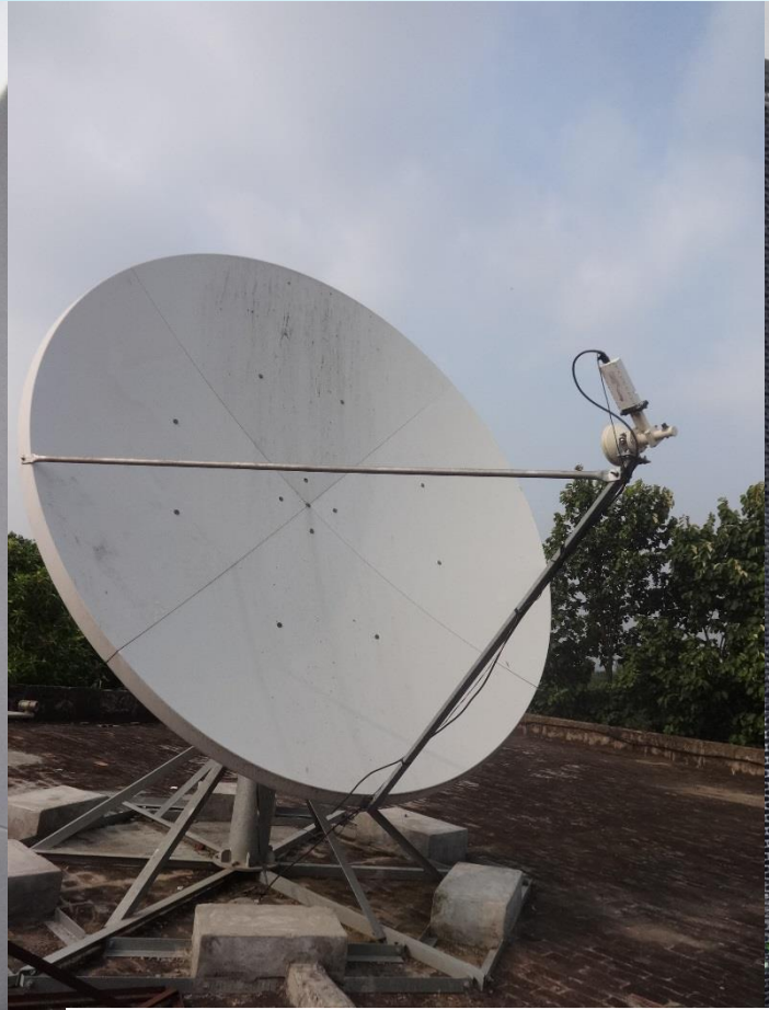
Dish on Rooftop
